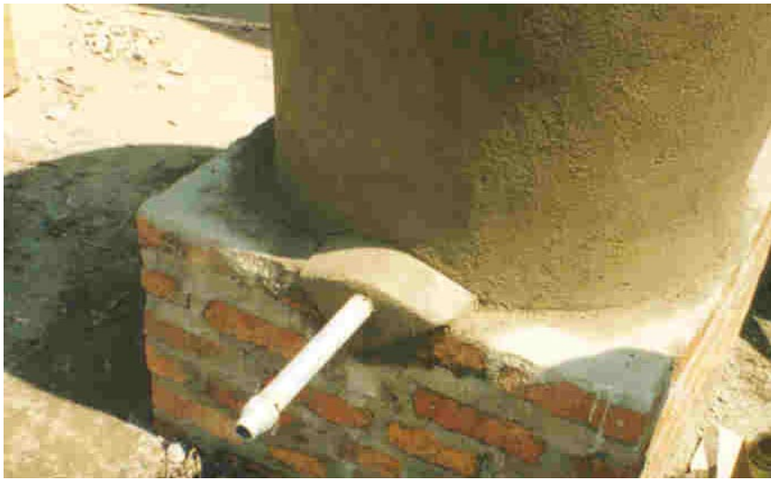
Figure 5 Detail of the outlet fixing
