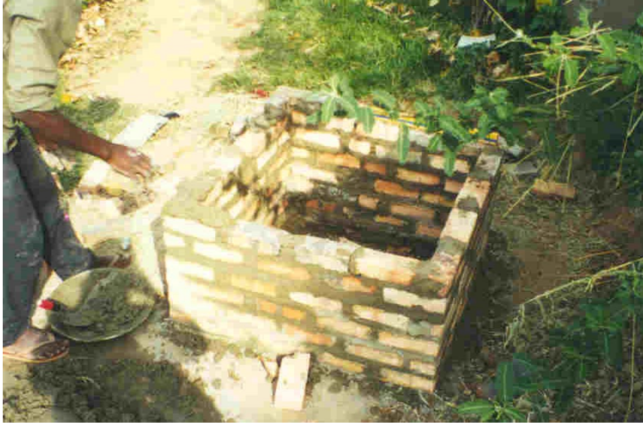
Figure 1 Brickwork plinth
